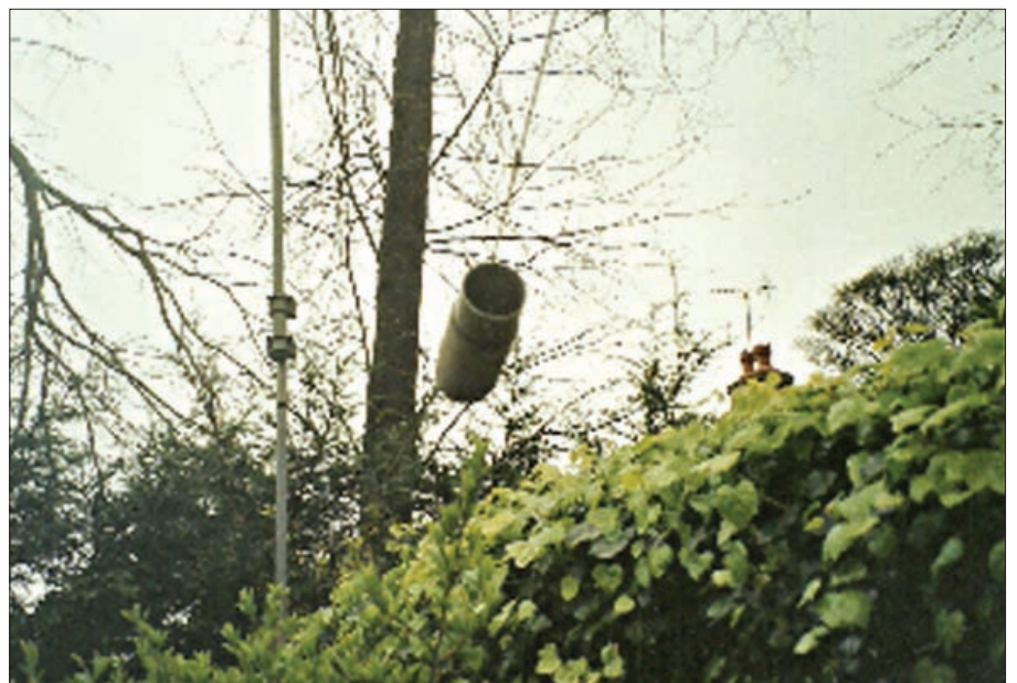
Fig. 4: The loading coil, L1 consists of 30 turns of antenna wire wound on a 50.8mm (2in) former and is placed 9.145m from the 'top' of the shunt coil. The outer end of the antenna has its length trimmed to give resonance of the whole system. As it might vary between about 9 and 12m a little experimentation will be needed. Some form of weather protection will probably be needed.
